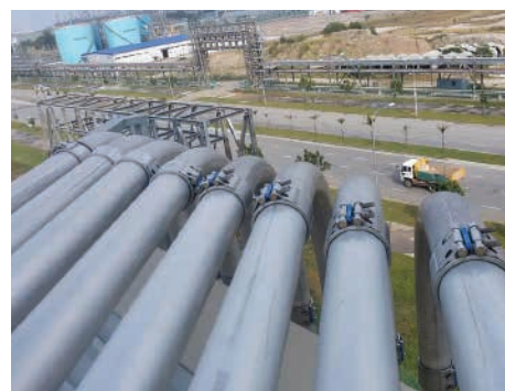
MJG. silo system.
