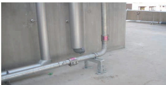
MJGF EPDM 50A. fire protection system. Japan
