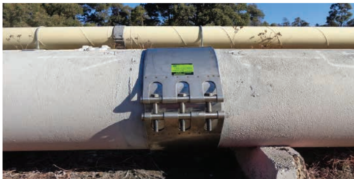
MJDL EPDM + strip insert 507mm. ash slurry line. 1km heavy weight fiberglass pipe of a coal fired power station. Australia
