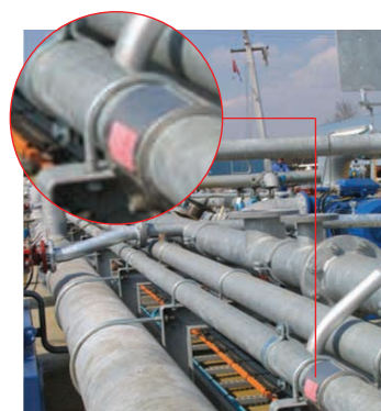
MJG EPDM 100A. sprinkler line for deck wash. Netherlands
