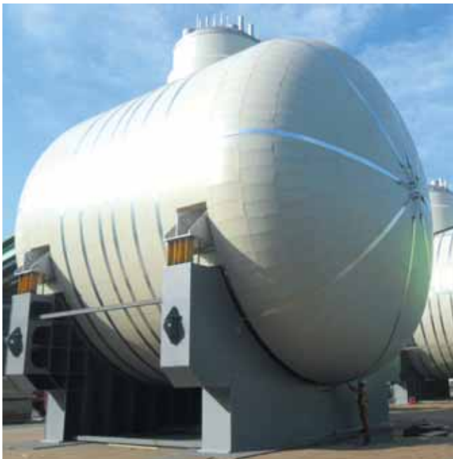
PMR & Ethane Tank Insulation for FLNG
