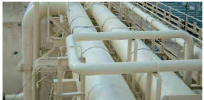
GRP Cladding Erection
