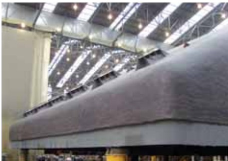
Upper Block Insulation
