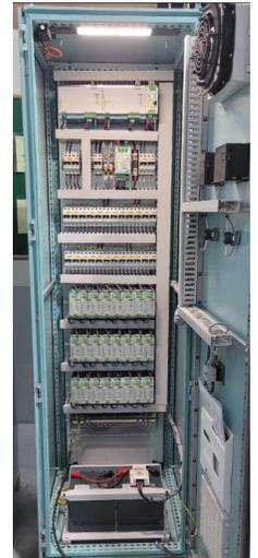
Interrupted Power Supply for ME Dual Fuel integrated ECS
