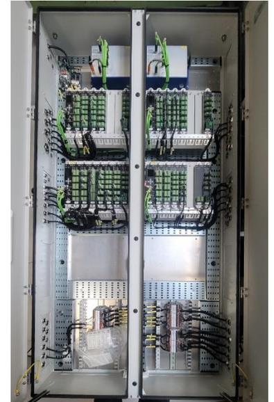
Engine Control System Cabinet / Cylinder Control System Cabinet / Second Fuel Engine Control Cabinet
