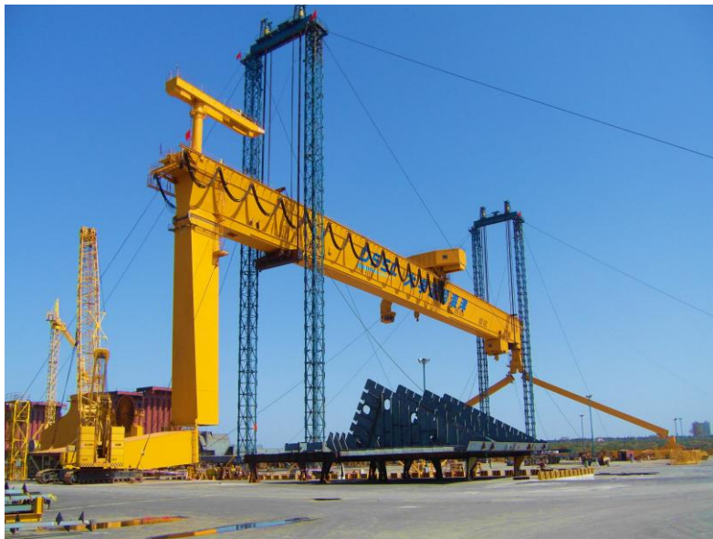
450t Goliath Crane Disassembling and Installation_DSME ( Korea to China Yantai )
