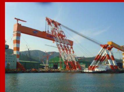
800 ton Goliath Crane Installation and Commissioning
