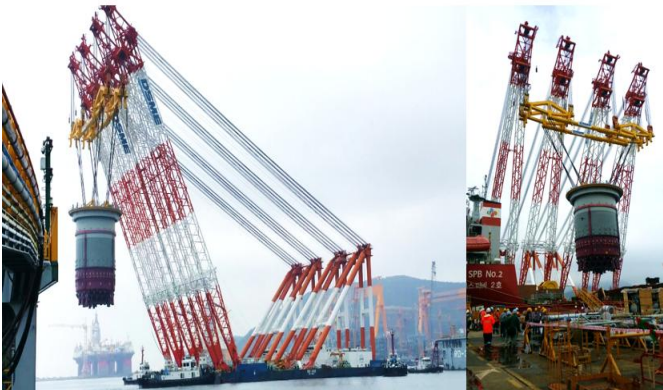
Dual Spreader Beam for 3,600 ton Floating Crane
