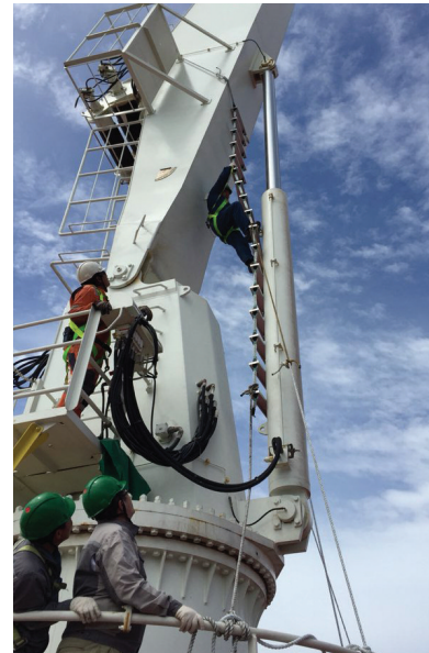
• Provision Crane Cylinder
